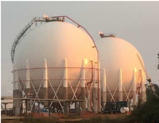
10 metre diameter Horton spheres storing extremely cold liquid hydrogen
