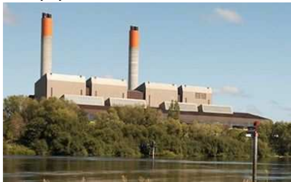
Genesis Energy’s Huntly Power Station is a thermal power station that can use coal, gas or both simultaneously as fuel. ( Radio NZ 14 Feb 18 )
